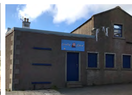
The Galley Shed
